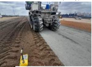
Recycler - Process of in situ execution of base and sub-base layers of pavements (recycled mixtures).
