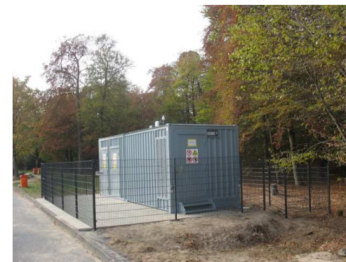
Rectifier substation and power electronics required every 1-4km
