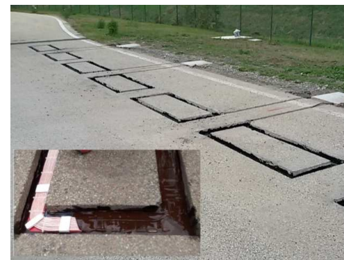
Trenched copper litz coils sealed in hot pour bitumen adhesive
