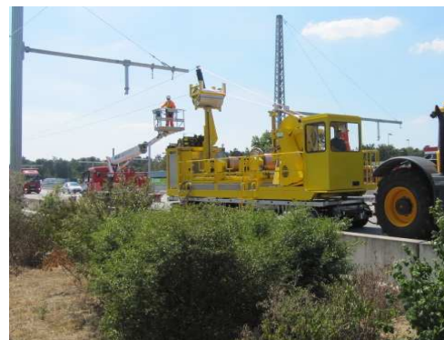
Copper cables fed through hangers and tensioned
