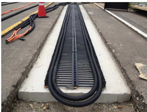
Trenched copper/litz coils with a ferrite core and concrete foundations with asphalt overlay
