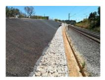
This intervention had the objective of improving the stability conditions of the excavation slope in the municipality of Soure, where there were several scars of landslides and ravines caused by erosion and water infiltration, guaranteeing the conditions of railway traffic in this section of track on which the maximum speed is 220 km/h.
