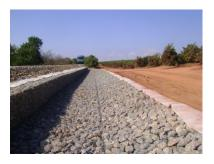
Actions developed with a view to stability, extension of the useful life and guaranteeing the safety of railway operation, under which the railway platform retaining wall was rehabilitated and reinforced, between km 388.395 and 388.560 of the Algarve Line, and an embankment stabilised with the extension of a gabion wall, between km 225.372 and 225.403 of the South Line.
