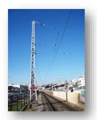
These works viewed to repair and paint overhead line posts in this railway line which is adjacent to the sea, and therefore exposed to significant deterioration and corrosion.
