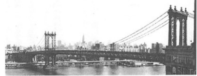
Manhattan Bridge will be stiffened by turning outer decks into torque tubes (shaded).
